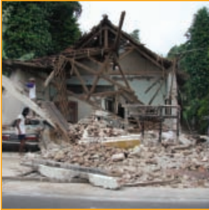
Collapsed buildings/rescue work
